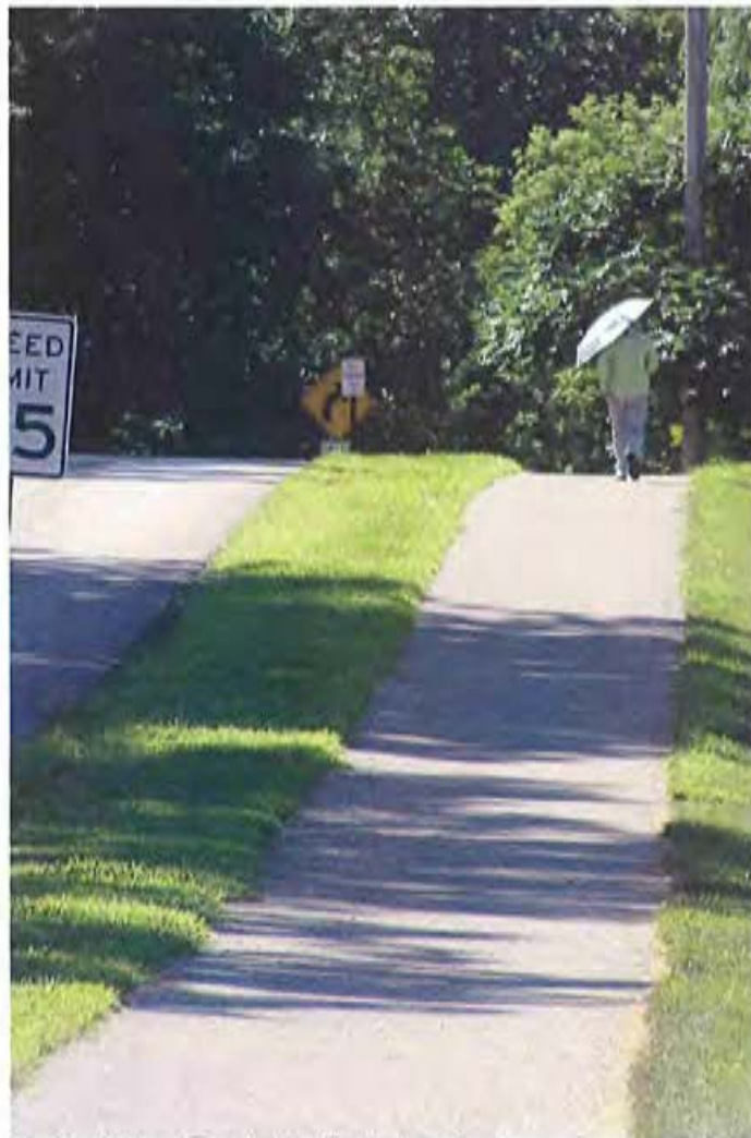
Six-foot bituminous trail - Covington Road
