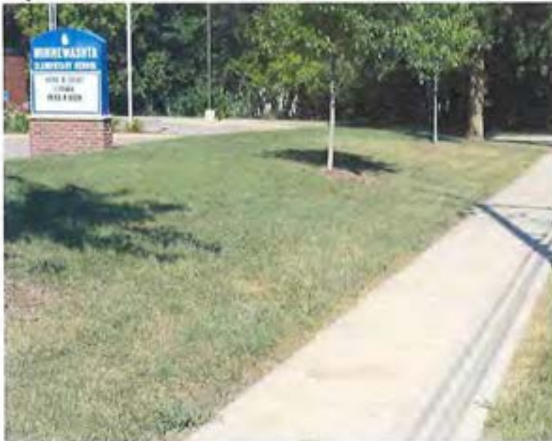
Five-foot concrete walk - Minnewashta Elementary
