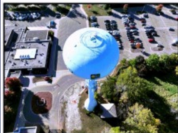
WATER TOWER, VIEWED SOUTH
