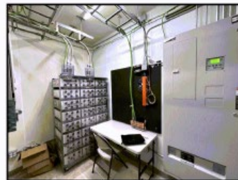
SHELTER, VIEWED NORTHEAST
