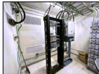
SHELTER, VIEWED NORTHWEST
